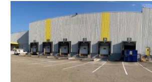
ID LOGISTICS 27 140 m 2 Saint-Quentin-Fallavier
